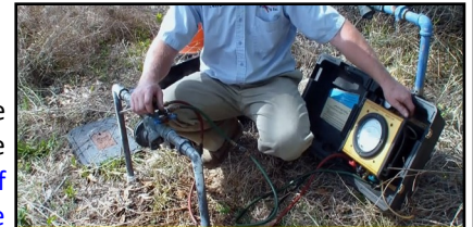
Testing a Backflow Device
